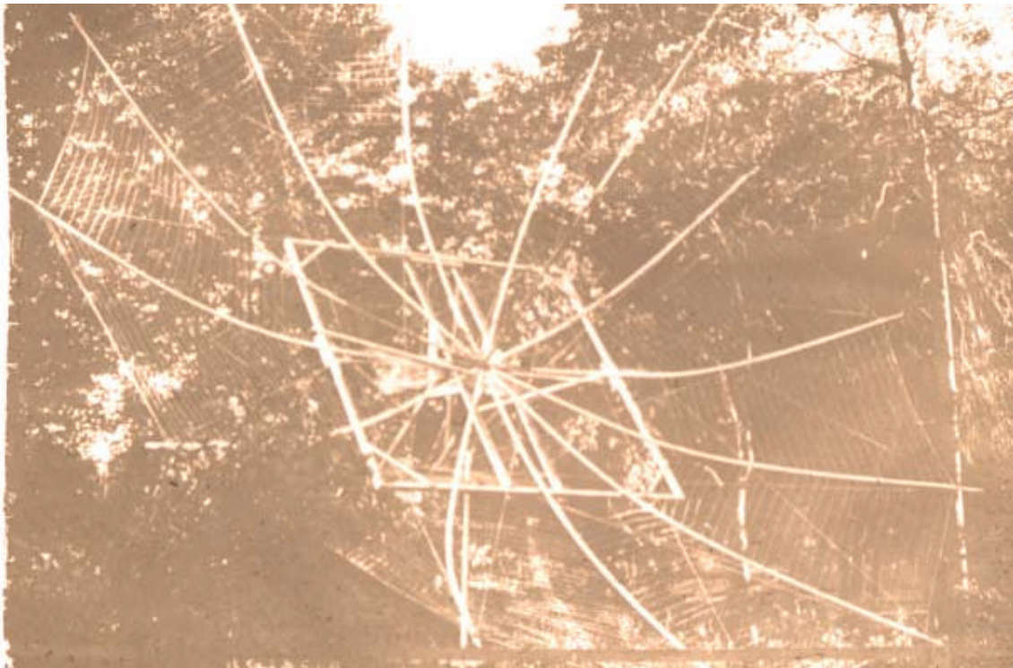
Figure 11. First stress dish (30' diameter) constructed by K2UYH in 1960.
